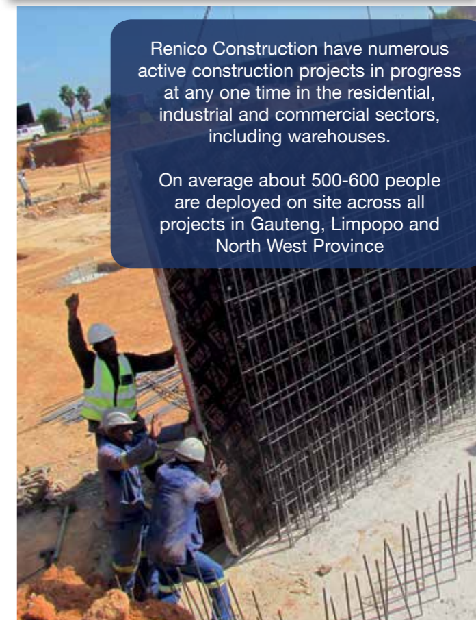
Peri formwork being hoisted into position
