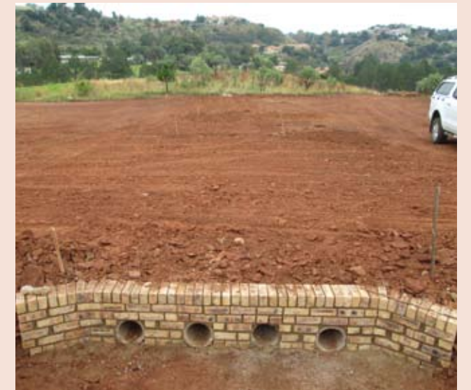
The "scorpion tunnel" at Ponders End
